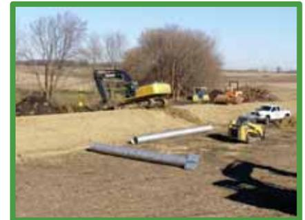
*Installing an earthen embankment and pipe to fix a gully entering Cobb Creek. Cost share provided by GBERBA and EQIP.*
