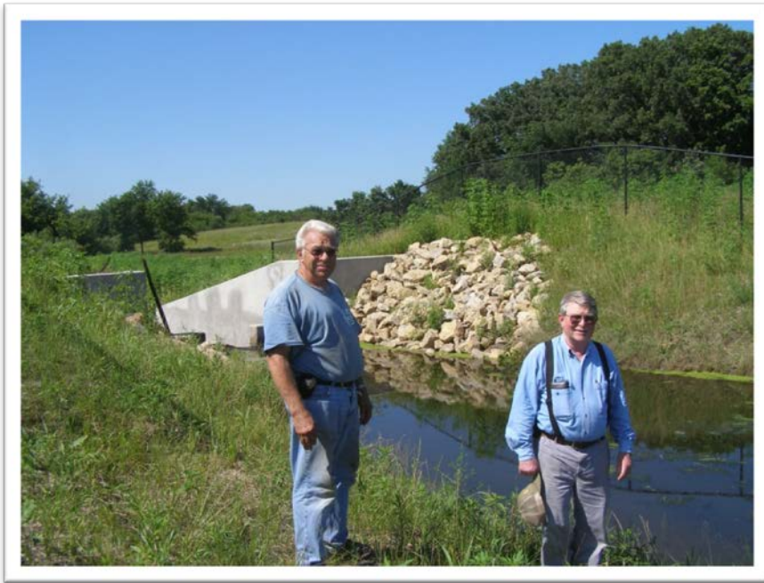
Large concrete water control structure
