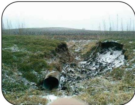
The Sept. rainstorm caused this damage to a Side Inlet Pipe along an open ditch. Flood Relief Funds can be used to repair these sites.
