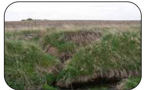
*This gully problem existed in the ditch bank prior to the installation of the new Side Inlet Pipe.*
