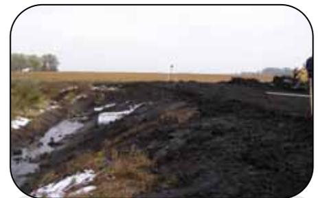
*Ditch bank now re-shaped and new pipes installed. Large pipe is for surface water and smaller pipe is for tile water.*
