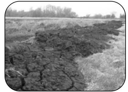
Sediment in drainage ditches is costly to remove and reduces capacity
